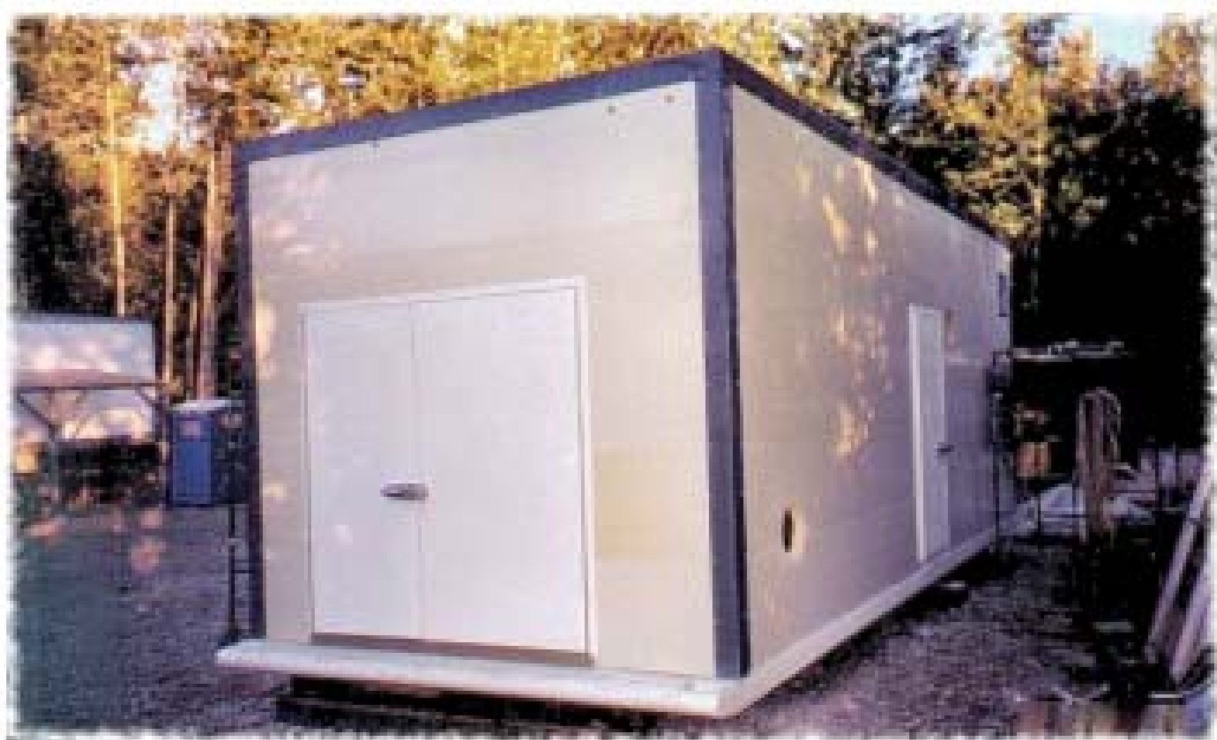
Modular Fuel Filtration Facility for U.S. Airforce, located in remote Alaska
